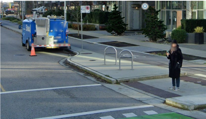
Concrete island on south side of East 1 st Ave, east of Quebec St, Vancouver
