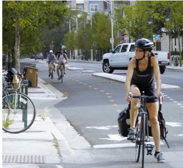
Concrete median adjacent to bi-directional cycle track; Rio Grande Street, Austin ( www.austintexas.gov/page/protected-bike-lanes )
