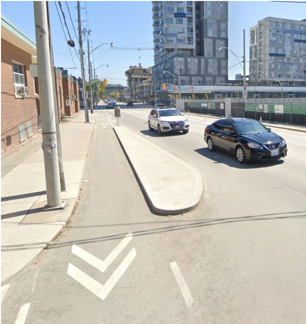
Concrete median adjacent to cycle track on east side of River St, south of Cornwall St, Toronto
