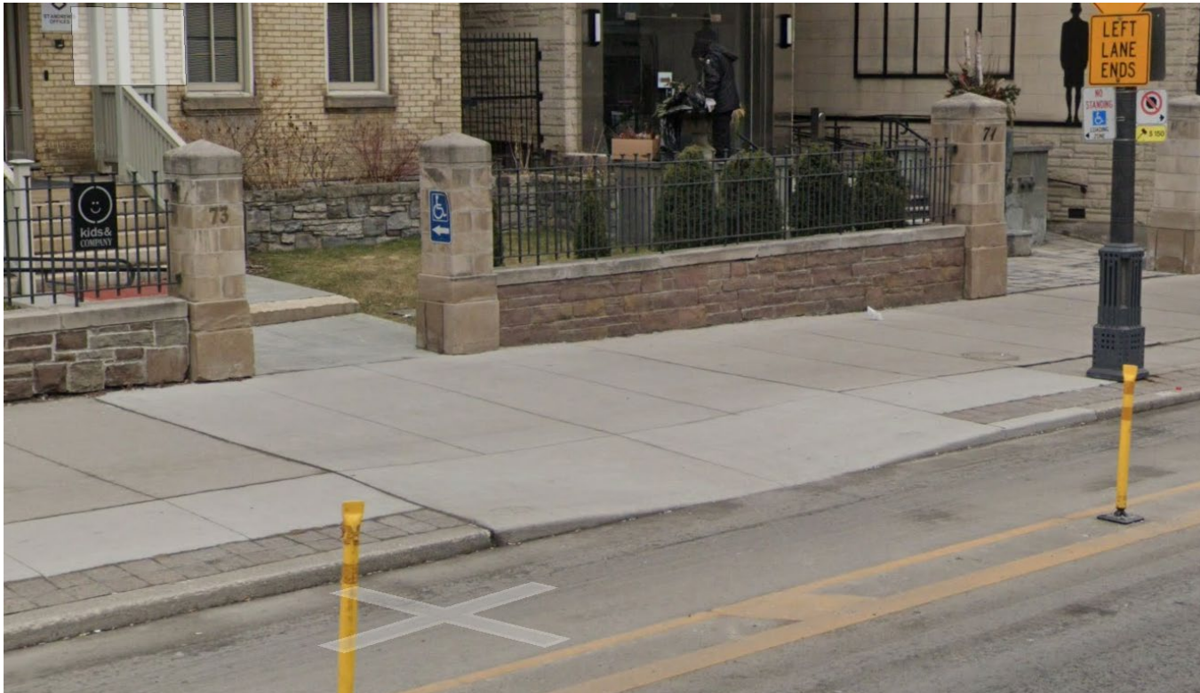
Dropped curb for St. Andrew's Church and office, east side of Simcoe St, south of King St West, Toronto
